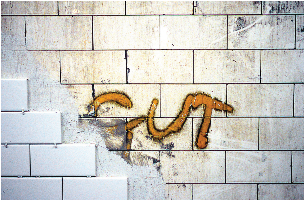
New tiling, NYC subway platform
